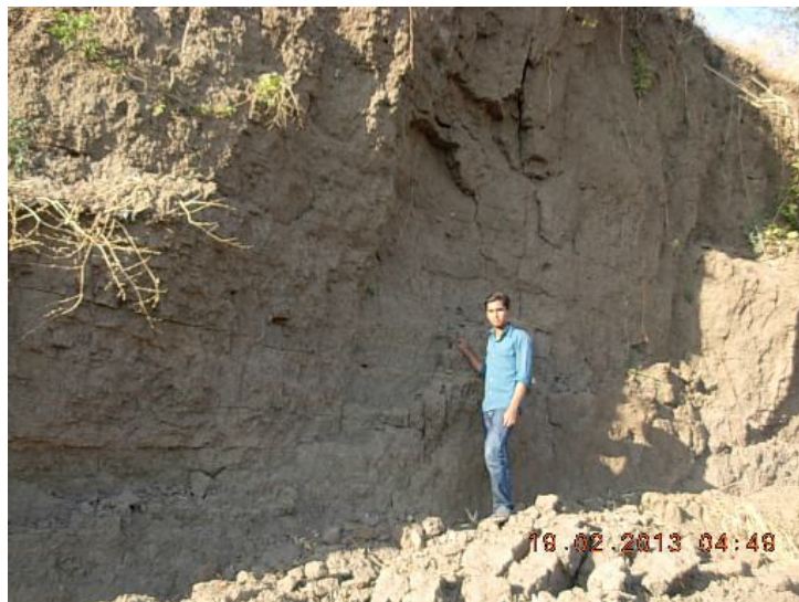
Fig. 4.12: Silty clay layers along left bank of Sindphana river at Nathapur
